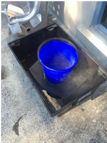
**Step 2** - Boil a kettle and place the pad in a plastic container for 5 minutes with the boiling water. This will allow the pad to be malleable and able to be shaped to the seat. The pad will need to be weighted down (eg use a bucket of water as a weight). NOTE: Failure to do this step may result in the pad cracking.
